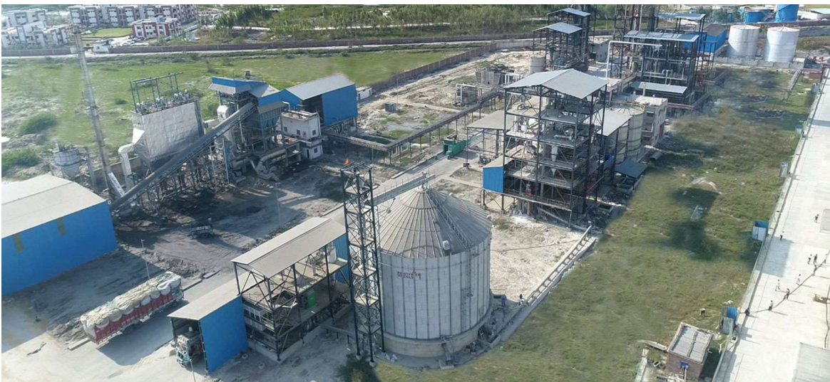
Sandila Plant, Dist Hardoi (U.P.)
